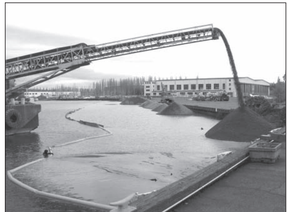
Placing gravel for new boat ramp and beach Photo courtesy of Seattle Parks and Recreation
